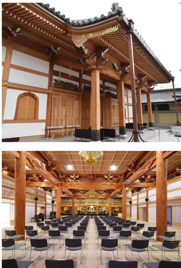
**Fig. 1** Keyaki wood used in traditional temple construction (Shogo-ji Temple, Miyazaki, Japan). Keyaki was used for main columns, beams with carving, and block and bracket clusters called Tokyou at the top of the columns
